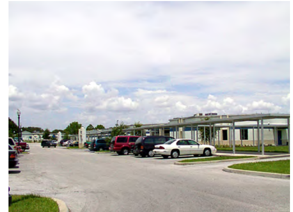
Figure 2.1 - The Beaumont development site currently provides poor pedestrian connectivity.
