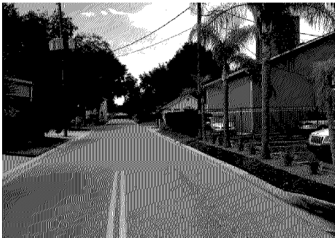
Missing sidewalks E. Walnut St.
