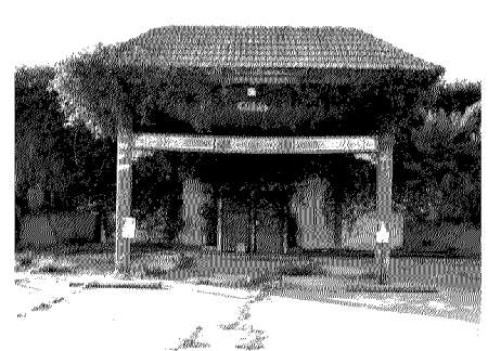
Completely deteriorated property.
